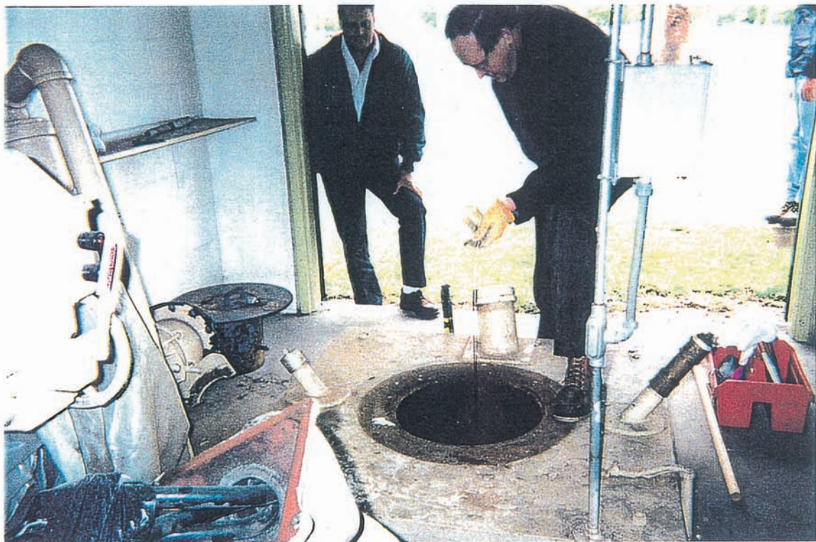
Lowering Coupons In Well No. 7
